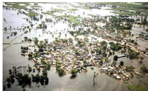
Picture 16 - Flooding in Operational Area
