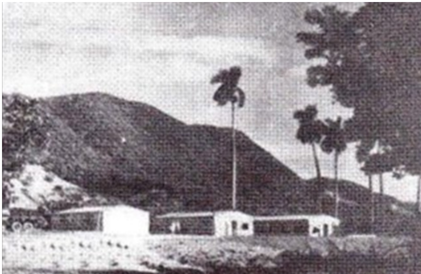
Figure 6 – Lodging for officers in modular structures
