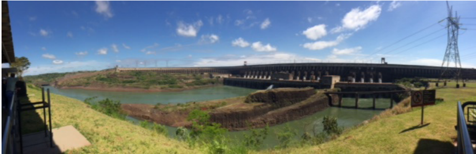
Figure 2: ITAIPU Dam is an effective example of world-class engineering skill coupled with Brazilian (& Paraguayan) efforts to harness social benefits through effective utilization of natural resources.
