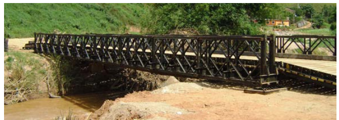
Fig. 2 – Double-simple Bailey bridge. Source: [4].
