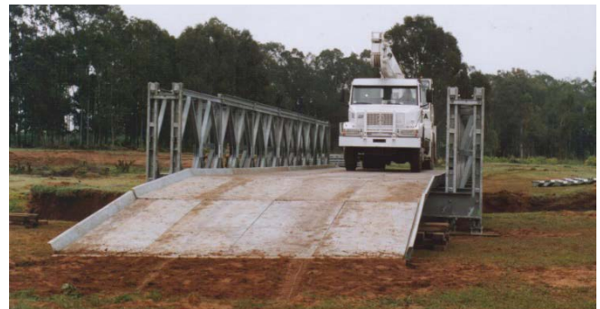
Fig. 8 – Compact 200 double-simple bridge. Source: [6].
