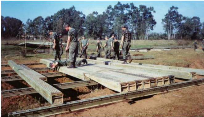
Fig. 6 – M4T6 bridge during assembly. Source: Authors' collection.
