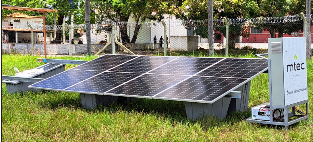
Figure 6 – Module 2: Campaign Energy Module on solar ballast (example with four modules)
